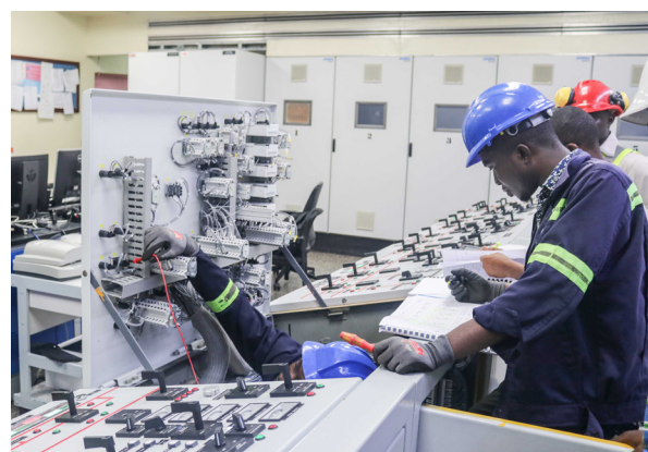
Technician engineers on duty.
